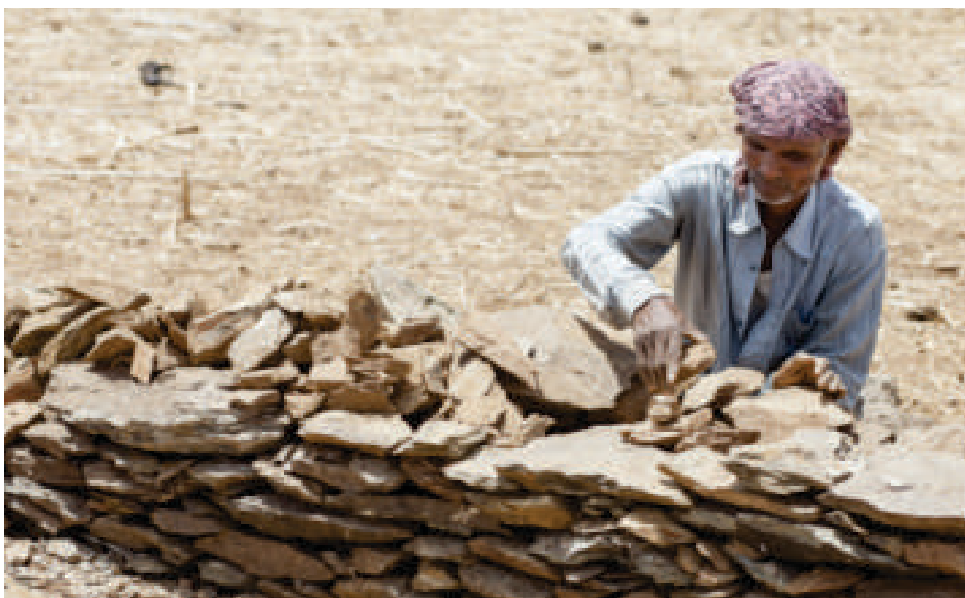
Protecting the commons by building a boundary wall, Jhadol Block
