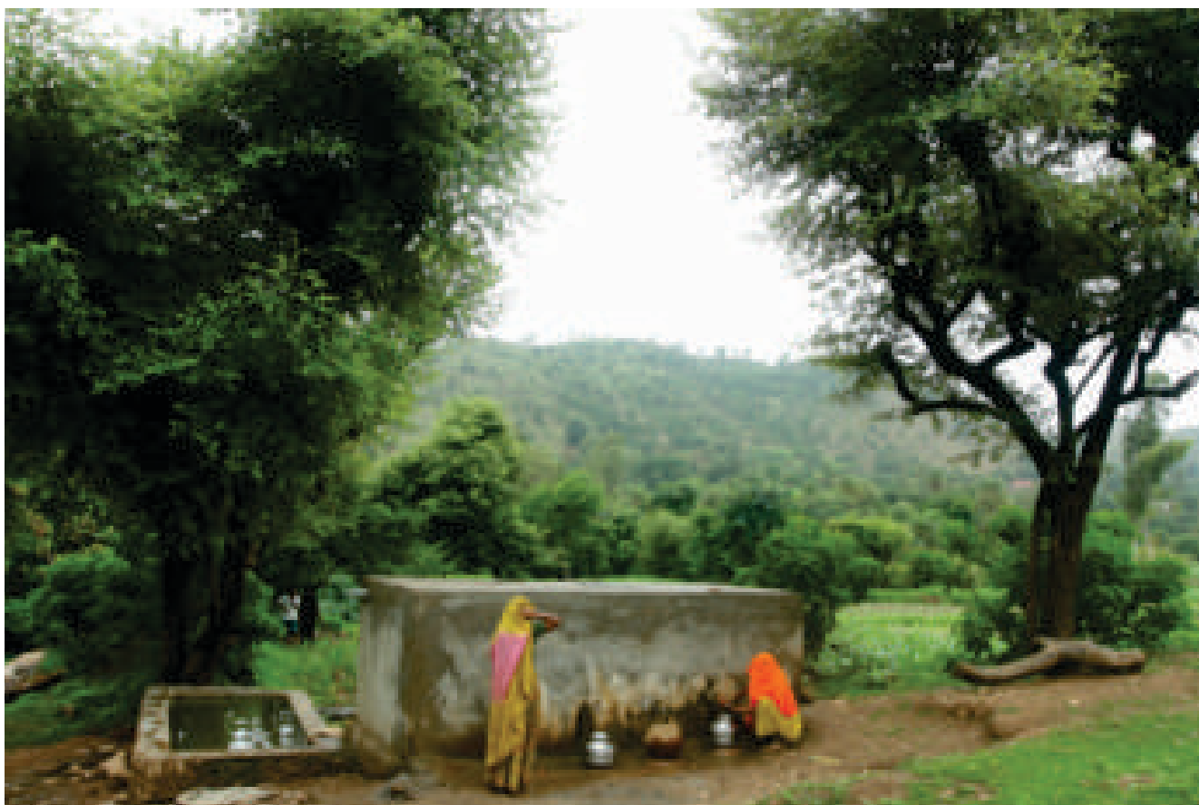
A closed water tank providing clean drinking water, Jhadol Block
